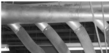
Multi-Tap Manifold (4 taps) for a sander used in a custom cabinet facility.
