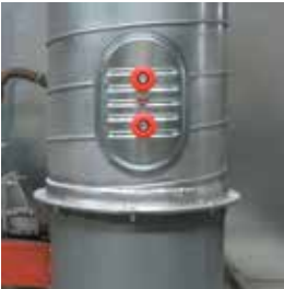
EASY Installation - Stick pattern on duct. Cut around pattern. Insert Door.
