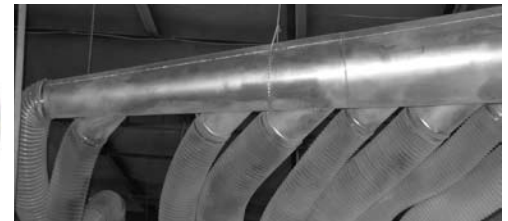
Multi-Tap Manifold (7 taps) for a sander used in a cabinet door facility.
