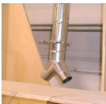
Light Gauge 45 Degree Y Branch with large end coupling making fitting to fitting connection between the Y Branch and Blast gate.
