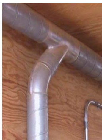
Light Gauge 45 Degree Elbow, shown with Lateral Tee and Spiral Pipe.
