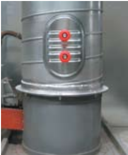
EASY Installation - Stick pattern on duct. Cut around pattern. Insert Door.
